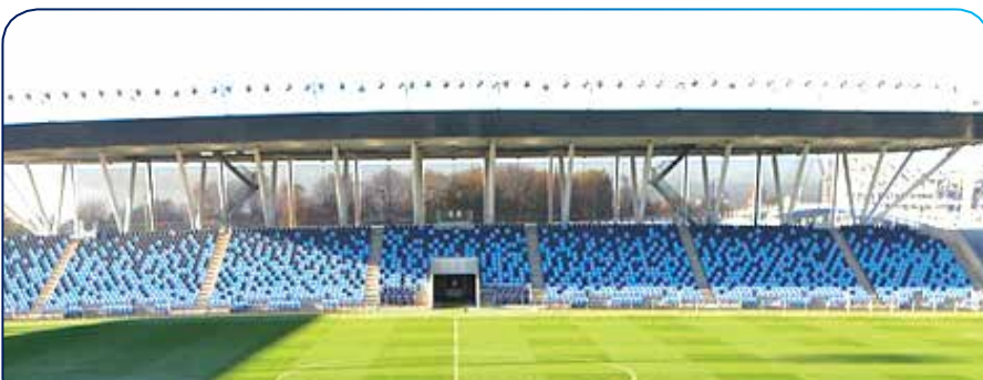
Figure 52. Example of a mini-stadium (International)
