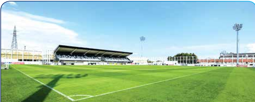
Figure 51. Example of floodlighting (International)
